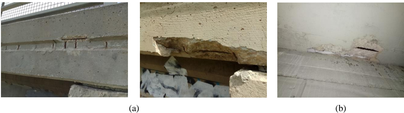
Fig. 8- Corrosion damage to bridge decks
