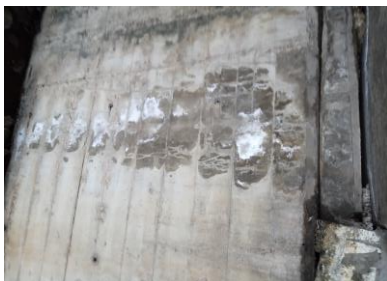
Fig. 10- Efflorescence damage to bridge elements
