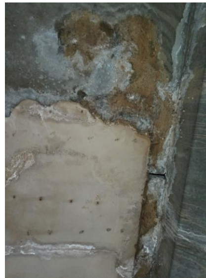
Fig. 10- Efflorescence damage to bridge elements
