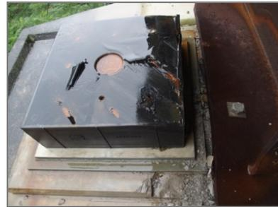
Fig. 5 – Failure of P4 pier G5 bearing
