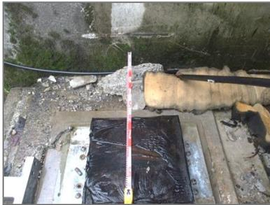
Fig. 4 – Failure of A1 abutment G5 bearing
