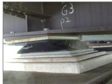
Fig. 7 – Failure of P2 pier G3 bearing
