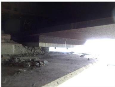
Fig. 6 – Failure of P4 pier G1 bearing
