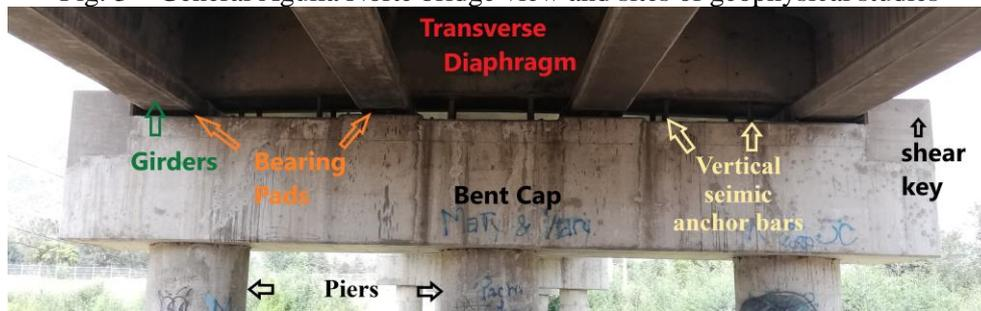
Fig. 4 –View of bent cap and connection between bents and the superstructure
