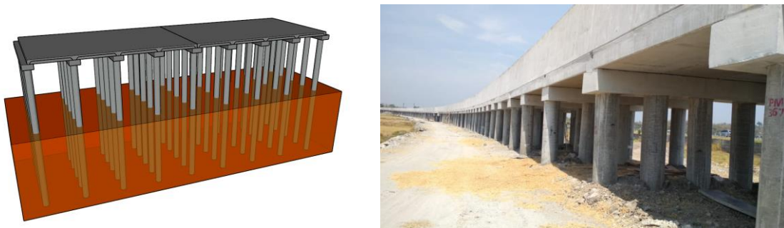
Fig. 1 – Typical configuration of pile-supported slab viaduct and the application in Adi Soemarmo Airport Railway Track
