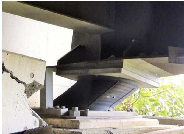
Photo 4(b) – Scratches on the upper shoe plate of A1G1 bearing (Mountain side)
