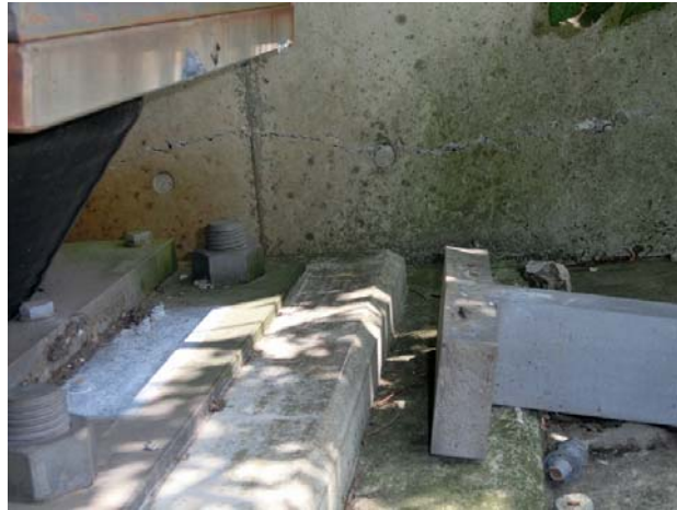
Photo 4(a) – Scratches on the upper shoe plate of A1G1 bearing (Valley side)
