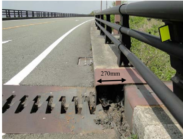
Photo 1 – Finger-joint device of A1 abutment
