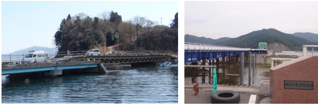
Fig. 6 – Temporary bridges constructed after the 2011 Great East Japan earthquake
