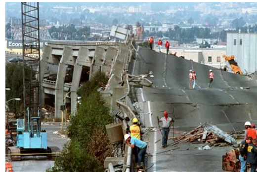
b) Damaged highway bridge in Loma Prieta
