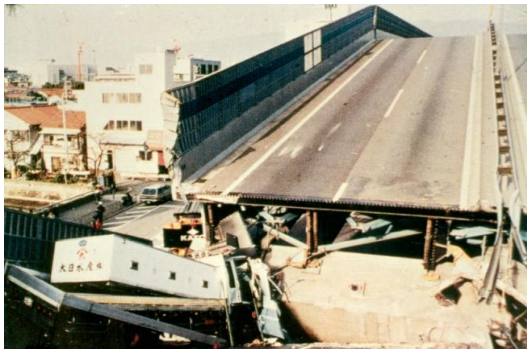
a) Collapsed bridge during Kobe earthquake
