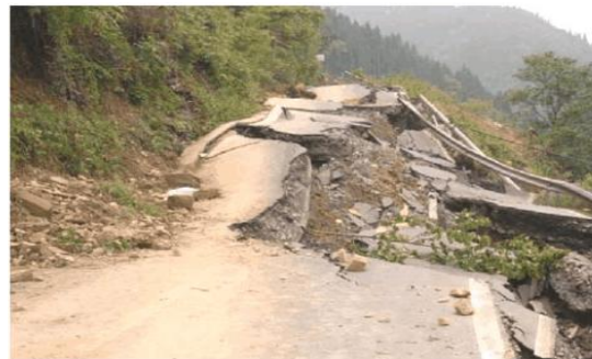
d) Damaged roads in Wenchuan earthquake
