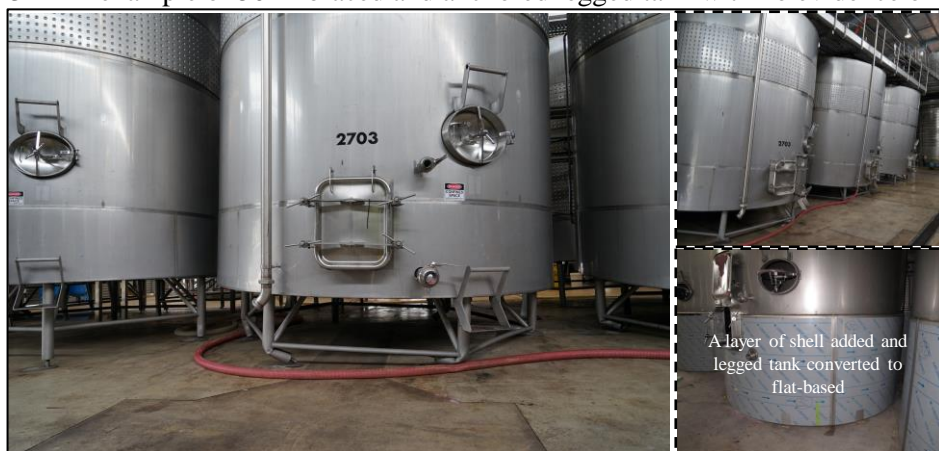
Figure 4 – Damaged legged tanks converted to the flat-based tanks following the 2016 earthquake
