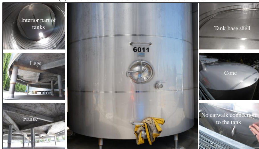
(b) Legged tanks and associated elements
