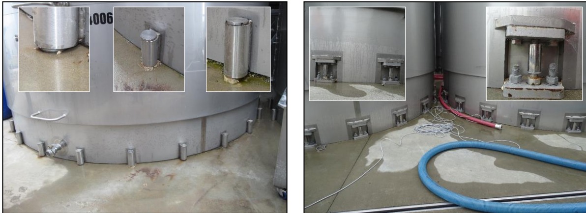
Figure 7 – Energy dissipation devices installed in wineries as part of resilience measures
