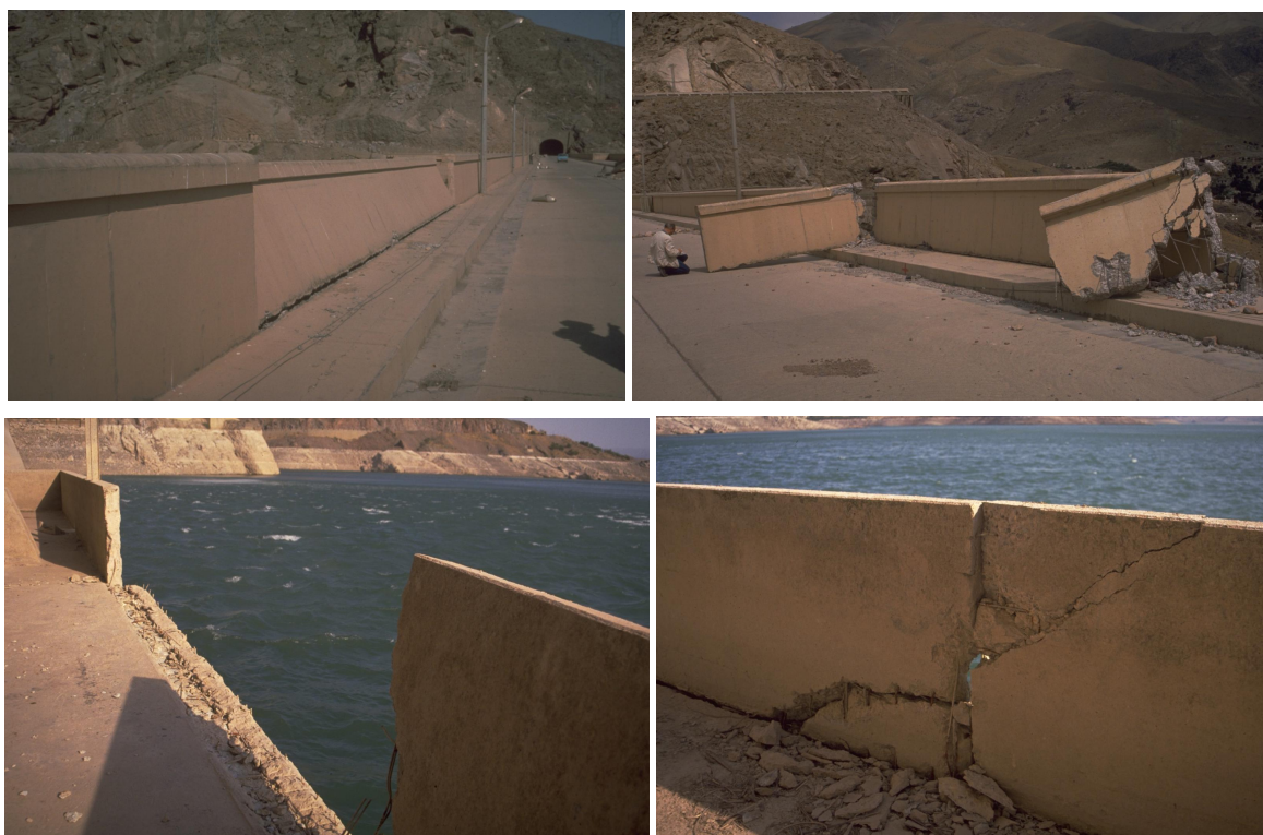
Fig. 6 – Tilting of concrete parapet wall on downstream crest (top left) and secured tilted wall after the earthquake to protect it from falling on the powerhouse (top right), damage at upstream face parapet walls above intake gates (bottom left and right)
