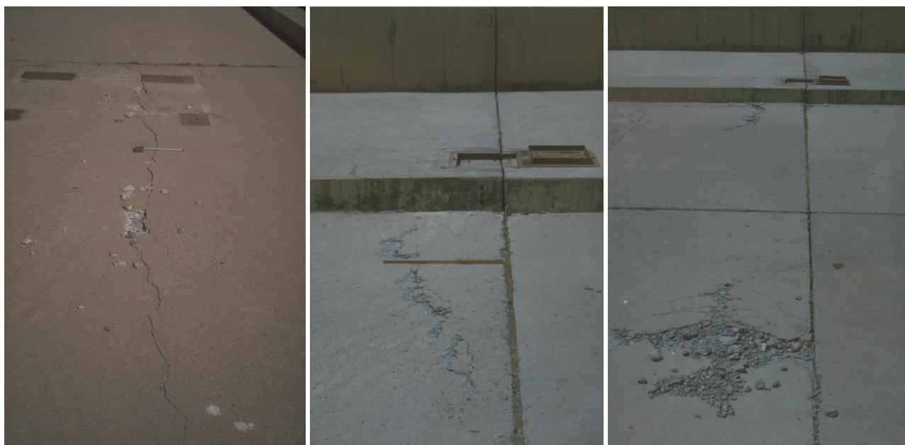
Fig. 5 – Cracks on dam crest due to high compressive stresses: Longitudinal crack (left) and compression-shear crack at block joints (centre and right) (Note: Relative movements occurred between some of the block joints)
