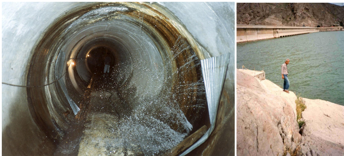
Fig. 10 – Leaking fissure in foundation gallery (left) and trace of fault of Manjil earthquake (right)
