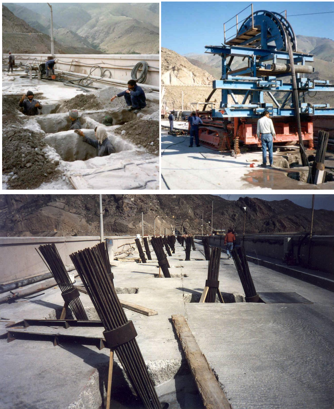
Fig. 17 - Repair work at Sefid Rud dam: Excavation for placement of anchor heads (top left), placement of anchor by homing device mounted on a crawler chassis (top right) and installed rock anchors before stressing (working load of each tendon: 8.4 MN) and final placement of anchor heads (bottom)
