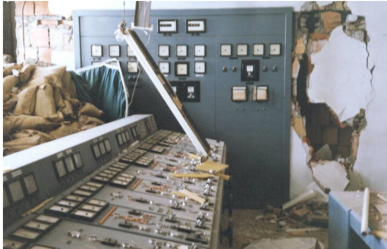
Fig. 12 – Damage in the control room of the hydropower plant caused by ground shaking (Note: The sandbags at the left were placed as protection from missiles as the dam and power plant were attacked by fighter planes during the Iran-Iraq war of 1980-1988)
