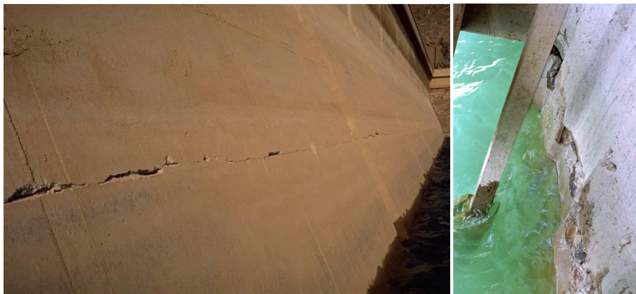
Fig. 4 – Horizontal crack at upstream dam face through several buttresses along lift joint (left) and horizontal crack and spalling of concrete above intake gates (right)
