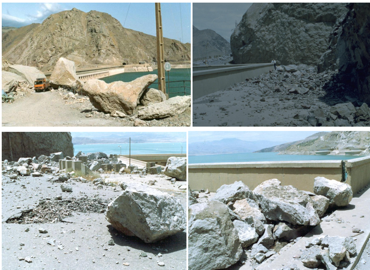
Fig. 11 – Rockfall at the dam site: Large displaced rocks above the spillway intake on left bank (top left)
