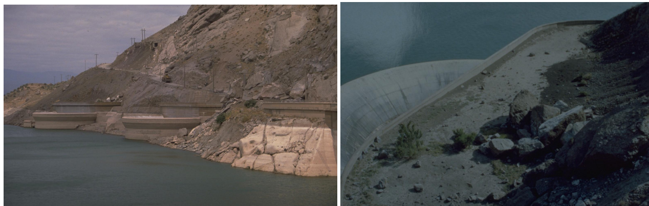
Fig. 7 – Rockfalls at intakes of morning glory spillways on left dam abutment: main rocks could be withheld by horizontal platform above intake (right)
