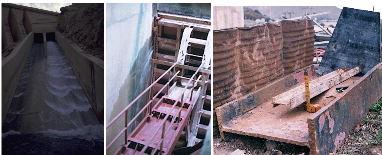
Fig. 8 – Damage of radial gate of intermediate level spillway causing leakage (left and centre) and deformed portion of spillway arm due to high hydrodynamic pressures (centre and right)
