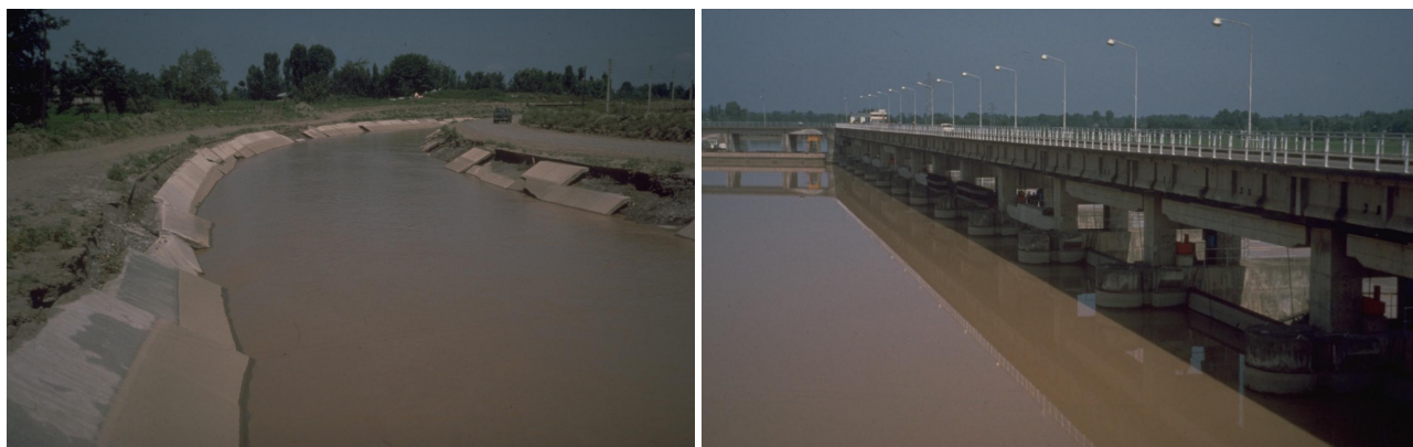
Fig. 9 – Damage of lining of downstream irrigation canal (left) and several counterweights for gate lifting of diversion structure of irrigation scheme were falling down (right)
