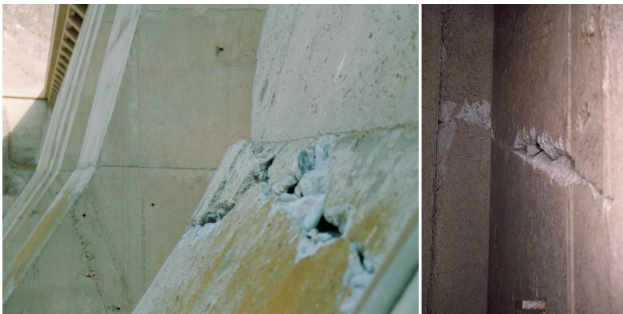
Fig. 3: Crack at kink location in buttress (left) and horizontal crack along lift joint (right)
