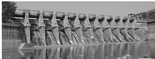
Photo 1 – Panoramic photo of the target facility
