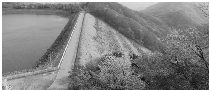
Photo 1 – Panoramic photo of the target dam
