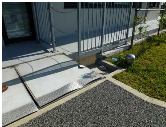
Fig. 8 A deformed gap cover
