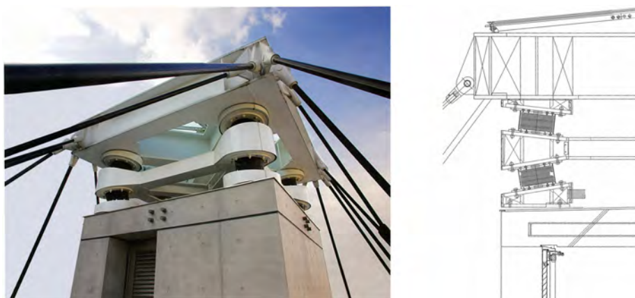
(b) Pendulum seismic isolation (SI) mechanism comprising two layers each of four inclined rubber bearings
