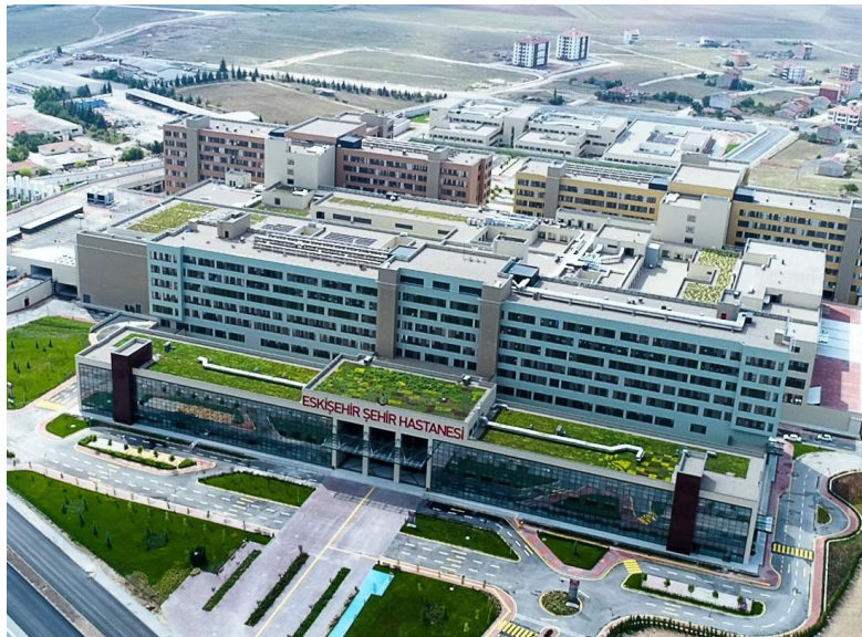
Fig. 1 – Eskişehir City Hospital issued by DOST Construction
