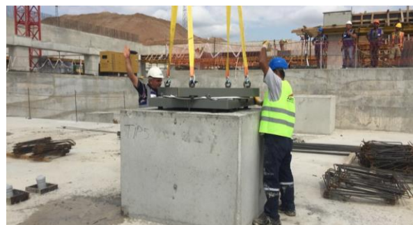
Fig. 11 – SIP D isolators ready for dispatch (left); positioning of isolator on plinth in the cellar level (right)
