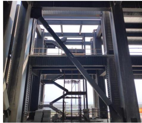
Fig. 18 Application of TYBRBs in Shanghai Tonghua Cold Warehouse
