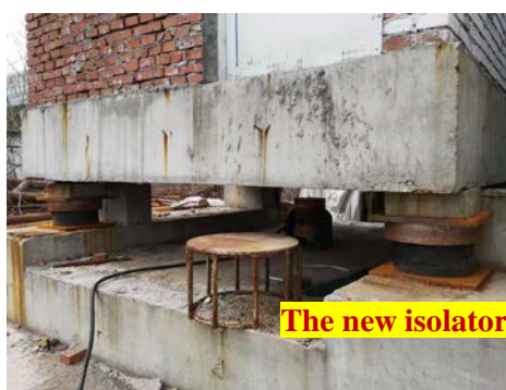
(c) The installed new isolator.
