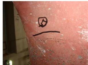
(b) The crack of arc segment (192mm)
