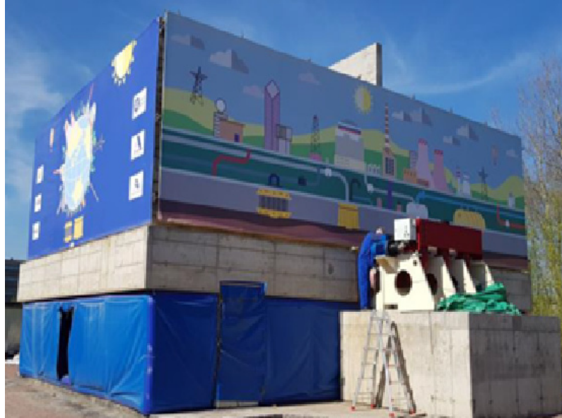
Fig. 5 – General view of the SIST
