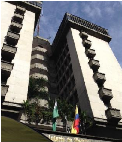
a) Building's frontal façade
