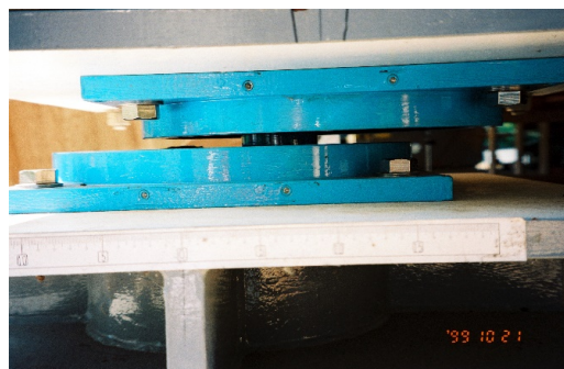
Photo. 2 – Displacement of isolator(no dust cover)
