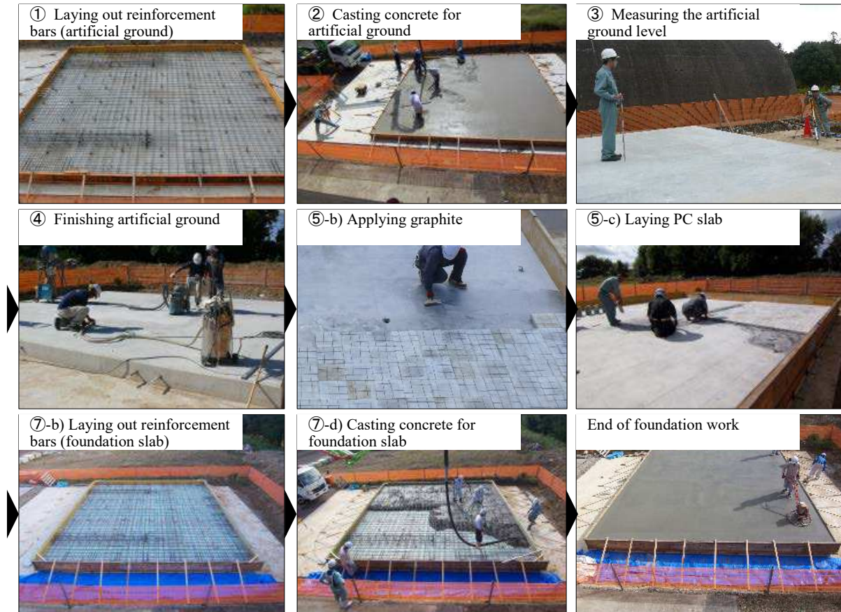
Photo 3 – Construct situation of full-size
