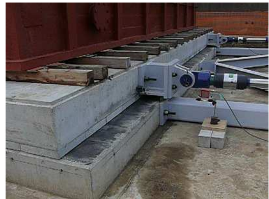
Photo 4 – Test implementation situation
