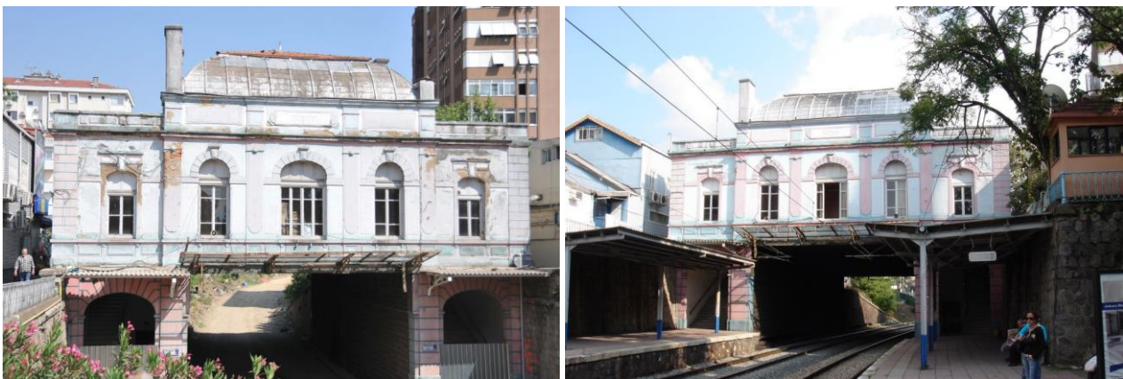
Fig. 8 – Recent Photographs of the Station Before Strengthening
