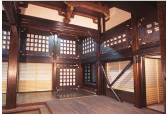
Photo 6 Large-scale wooden building (retrofit)
