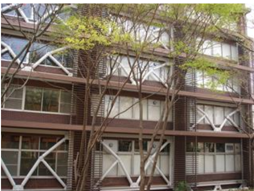
Photo 4 University of Tokyo (retrofit)
