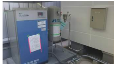
(c) Air pressure control system
