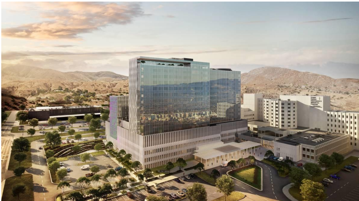
Fig. 1 – Architectural rendering of the replacement hospital with the SPC-1 cloverleaf building in the background ( Image: NBBJ )
