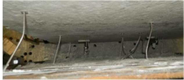
Fig. 22 - Wall ties after load level 2 up to  $V = 2$  kN
