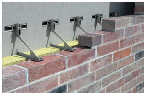
Fig. 2 – Example of brickwork support
