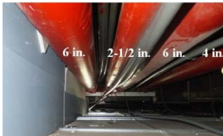
Fig. 2 – Piping layout in the corridor
