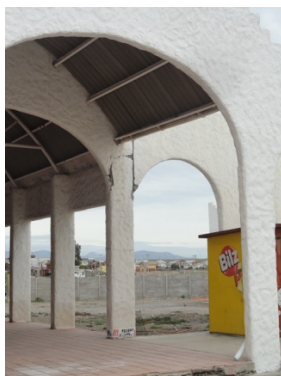
(a) Slight damage in some connections
