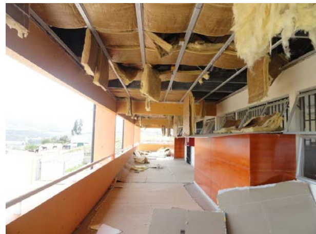
(b) Nonstructural damage of the ceilings
