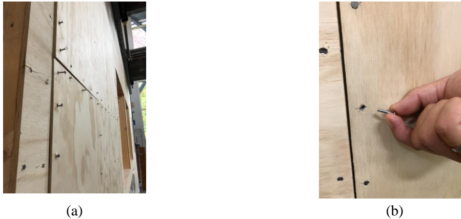
Fig. 7 - Damage in Specimen Sp-10 after test #2: a) South-west shear wall, b) Shear off nail
