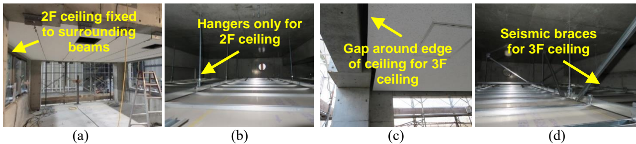
Fig. 5 – Ceiling detailing; (a) no gaps for 2F ceiling, (b) no seismic braces for 2F ceiling, (c) edge gaps for 3F ceiling, and (d) seismic braces for 3F ceiling
