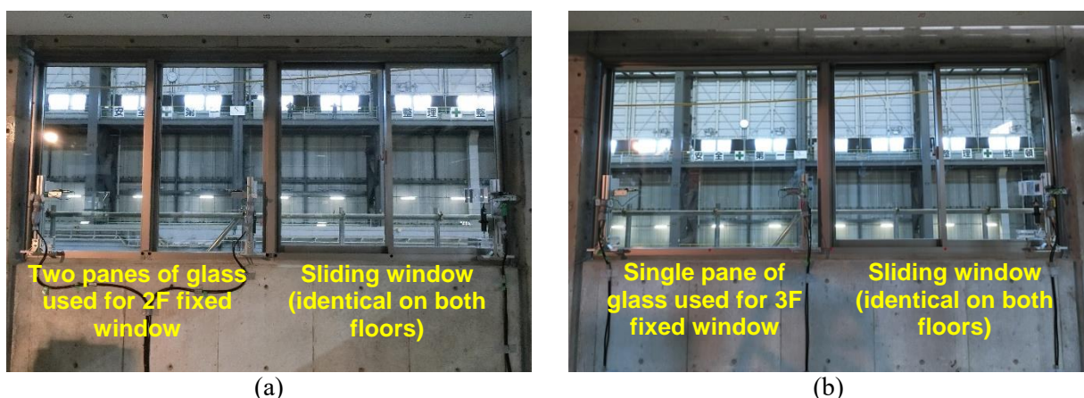
Fig. 4 – Window detailing; (a) two panes of glass used for 2F fixed window and (b) single pane of glass used for 3F fixed window
