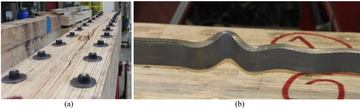
Fig. 10 – Failure modes: (a) specimen 2; (b) specimen 3
