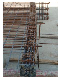
Fig. 3 – Anchorage setup for PC strands
