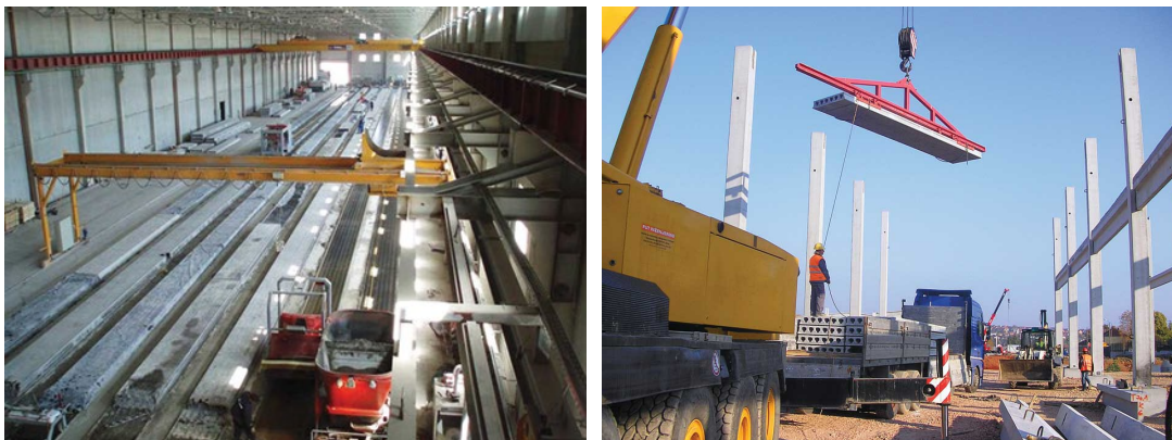
Fig. 2 Manufacturing and mounting of the precast prestressed hollow core slabs ( http://putinzenjering.com/about-us/?lang=en )
