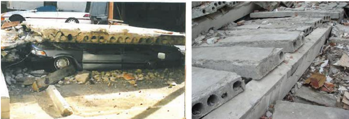
Fig. 1 Collapse of a complete section of floor, [6]
