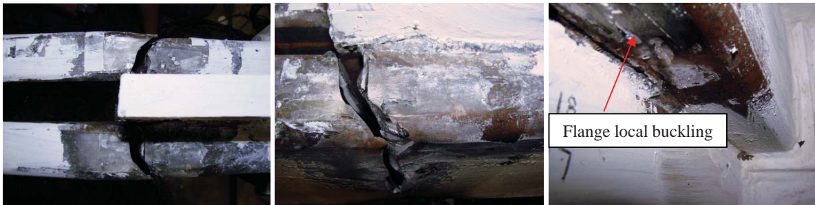
Fig. 7 – Fracture of link at the end of test (15% total rotation angle or 12% plastic rotation angle)
