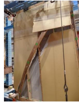
(c) N-side damage
