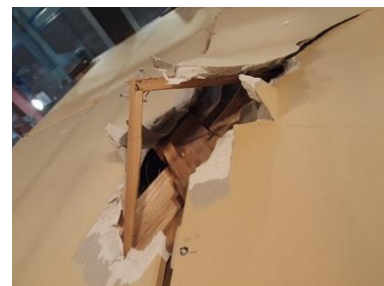
(c) Bracing damage (1/50 rad)
