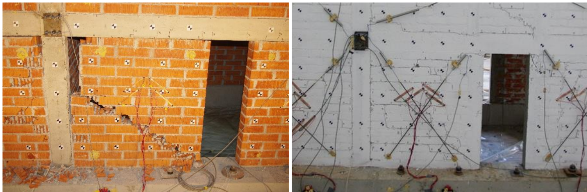
Fig. 10 – Observed damage to frame A on the first floor after the final tests in both series: (left) Series 1, (right) Series 2
