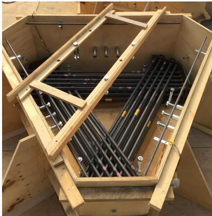
Fig. 4 – Photograph of formwork, reinforcement, and anchors for medium specimen.
