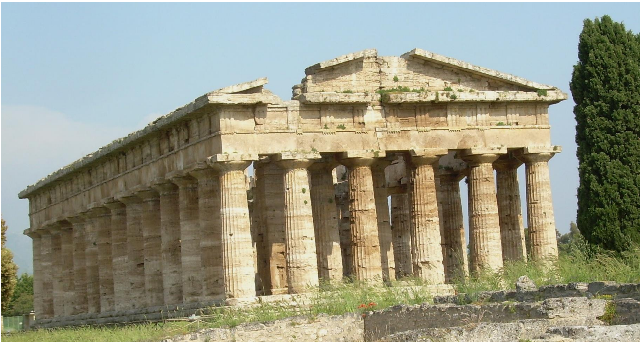
Fig. 1 – Temple of Neptune in Paestum, Italy, a world heritage site and reference structure for this project.
