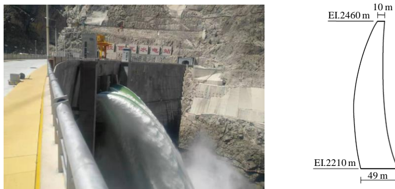
(a) dam (b) Cross-section of crown cantilever
