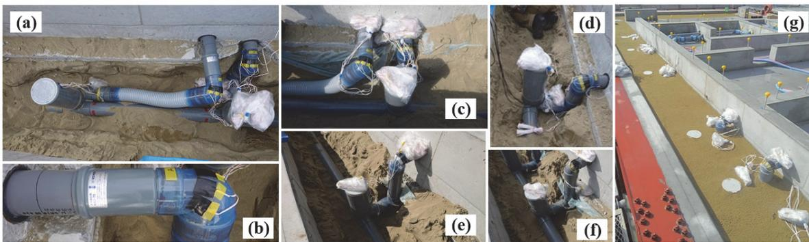
Fig. 5 – Placement of PVC drainage pipes
