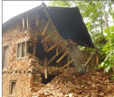
(b) Out-of-plane collapse of wall led to collapse of roof and floor, 2015 Gorkha earthquake, Nepal
