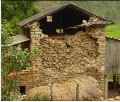
(a) Delamination and bulging of wall wythe, 2015 Gorkha earthquake, Nepal
