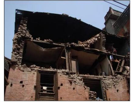
(c) Out-of-plane collapse of walls, destruction of top storey, 2015 Gorkha earthquake, Nepal
