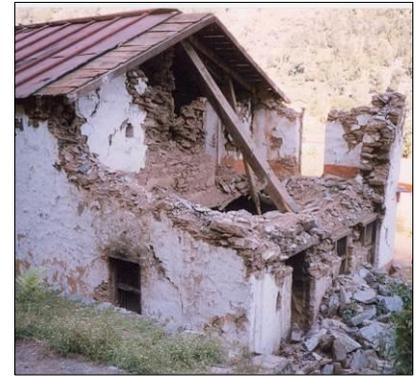
(f) Roof collapse due to absence of wall-roof connections, 1999 Chamoli earthquake, India
