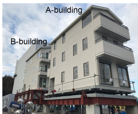
(1) Construction site (outside west yard)
