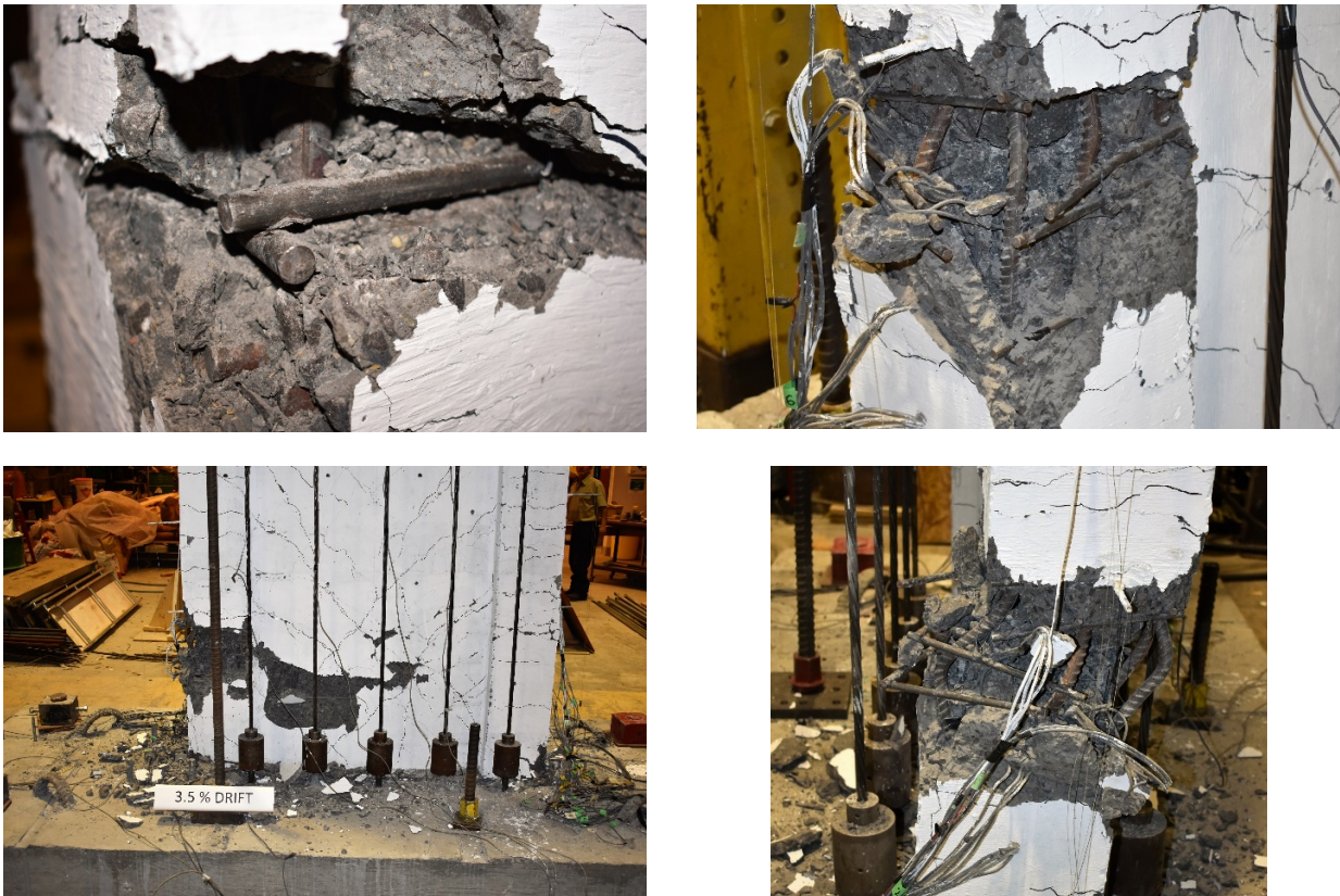
Fig. 10 – Shear wall at failure and observed damage to concrete and WWR grids
