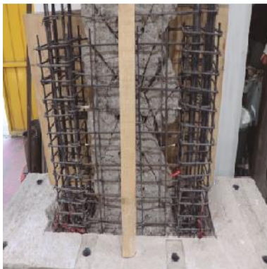
Reinstatement of new reinforcement
