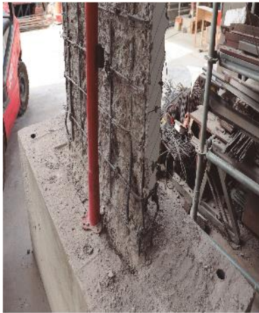
Demolition of concrete
