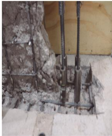
Use of anchors mechanic
