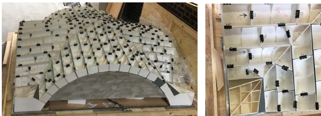
Fig. 11 - Pre-assembly of the plastic skin of the blocks.
