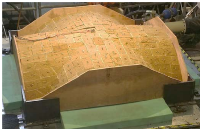
Fig. 15 - Wooden panels installed to provide confinement.
