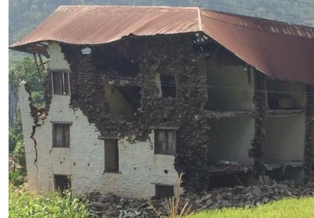
Delamination of the inner and outer walls
