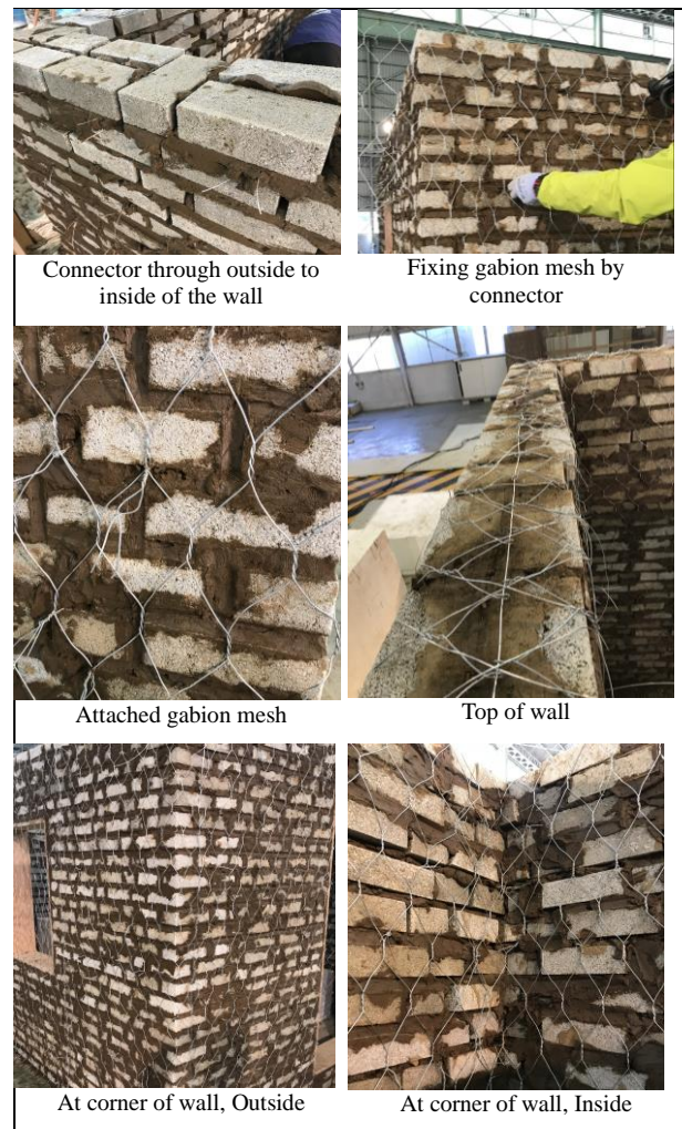
Fig.3-4 Installing gabion mesh
