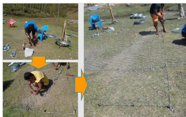
Fig.2-4 Installing gabion mesh on site
