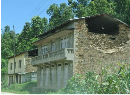
Gable wall failure
