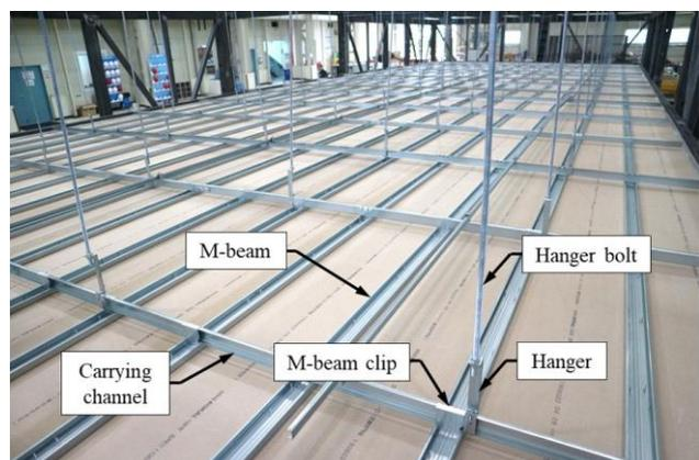
(d) Indirect hung suspended ceiling system (M-beam)
