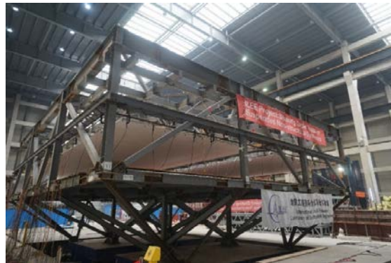
Fig. 1 – Overall view of the steel platform
