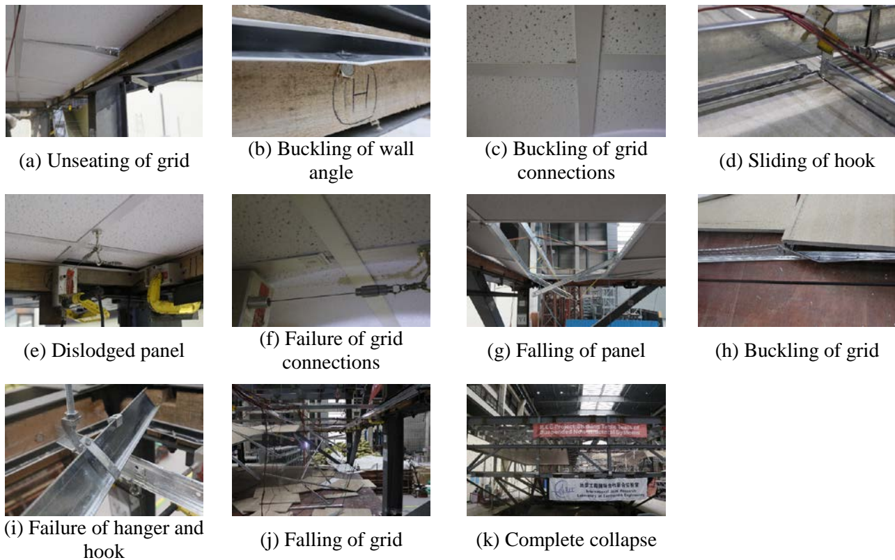
Fig. 5 – Failure process during test
