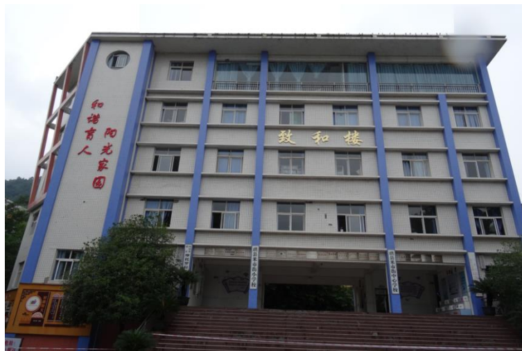
Fig.1 – Picture of the teaching building.
