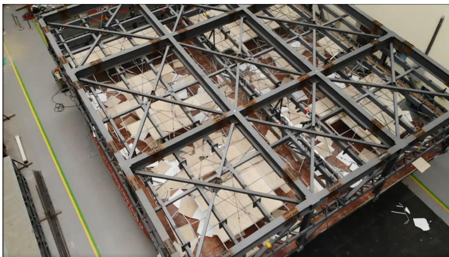
Photo 5 Ceiling experiments taken with a drone
